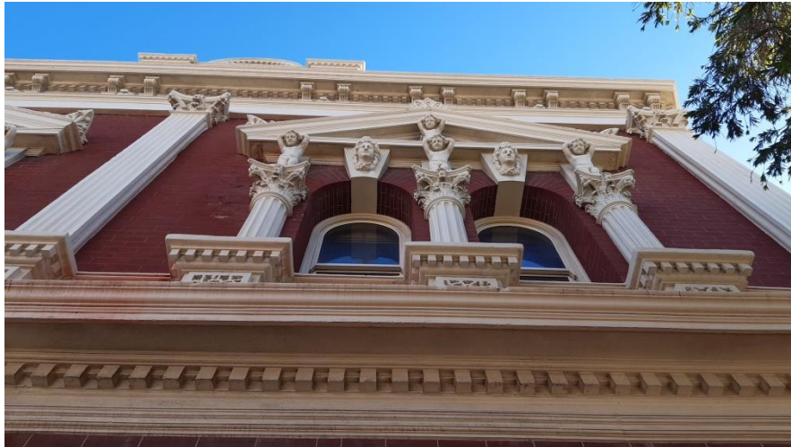
Glanville Building on Canning Highway
